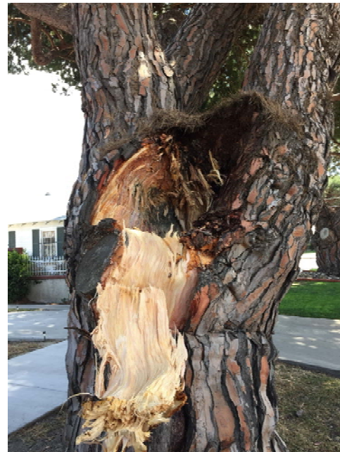
Note pocket of decay on the NE quadrant
