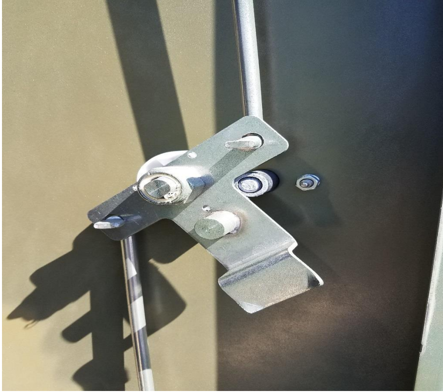
Figure 3 - Interior Configuration of Locking Mechanism
