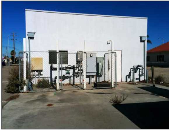
South elevation, view looking north.
