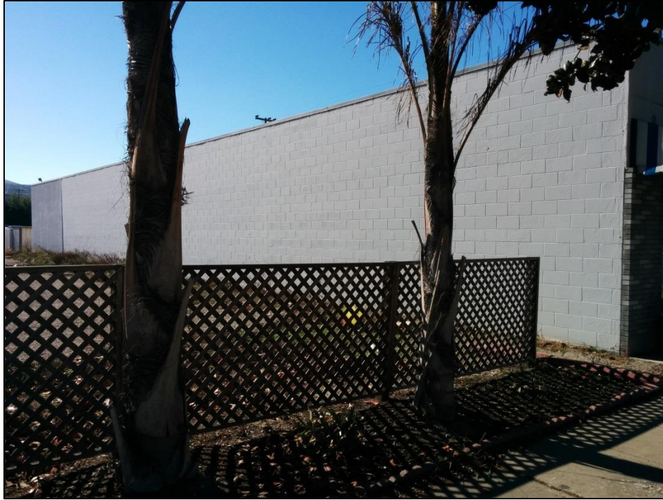
East elevation, view to the southwest.
