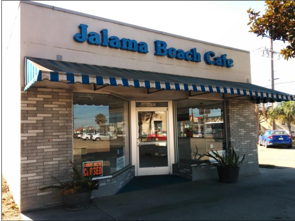
Northern façade, view to the southwest.
