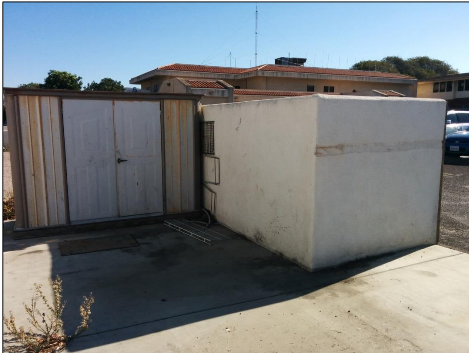
Storage shed and trash enclosure, view to the southeast.
