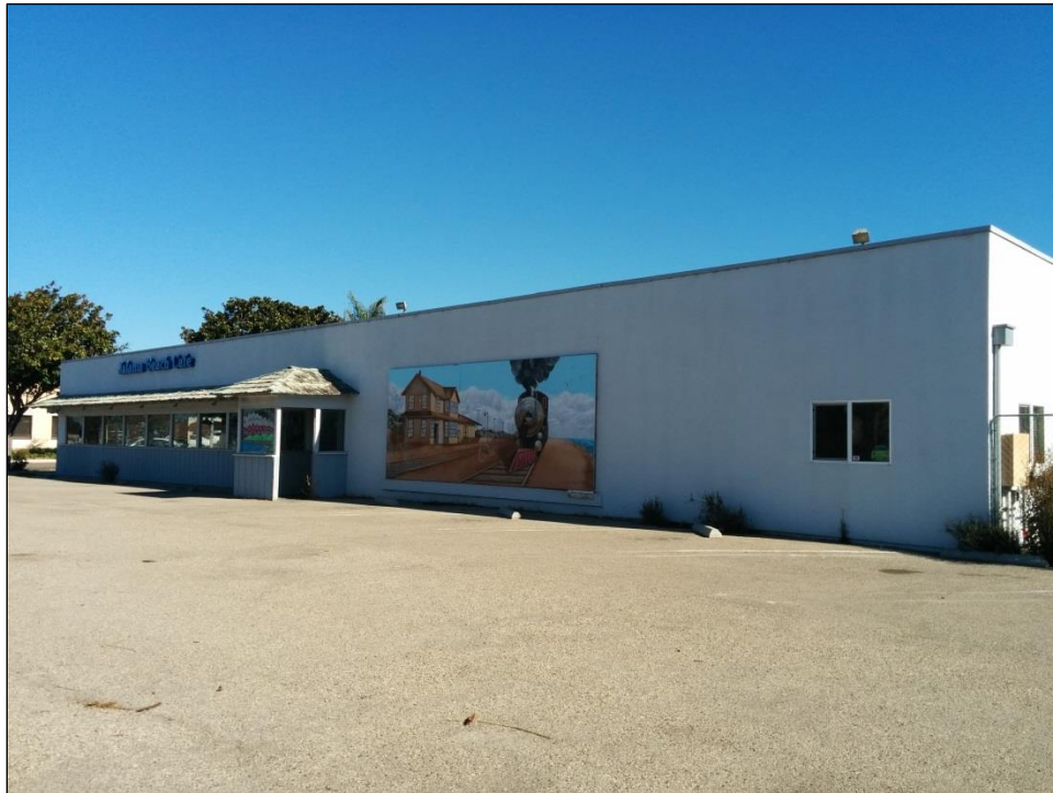
West elevation, view to the northeast.
