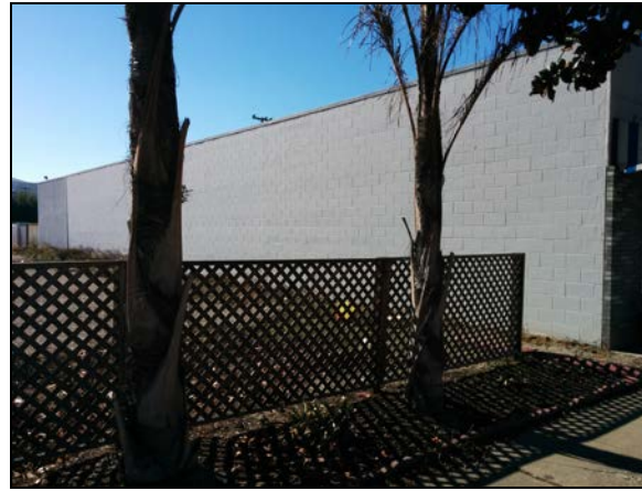
East elevation, view looking southwest.
