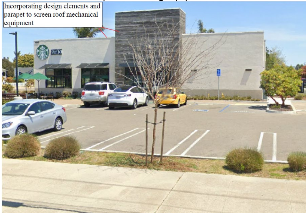
Picture Example: Screening equipment on the roof
