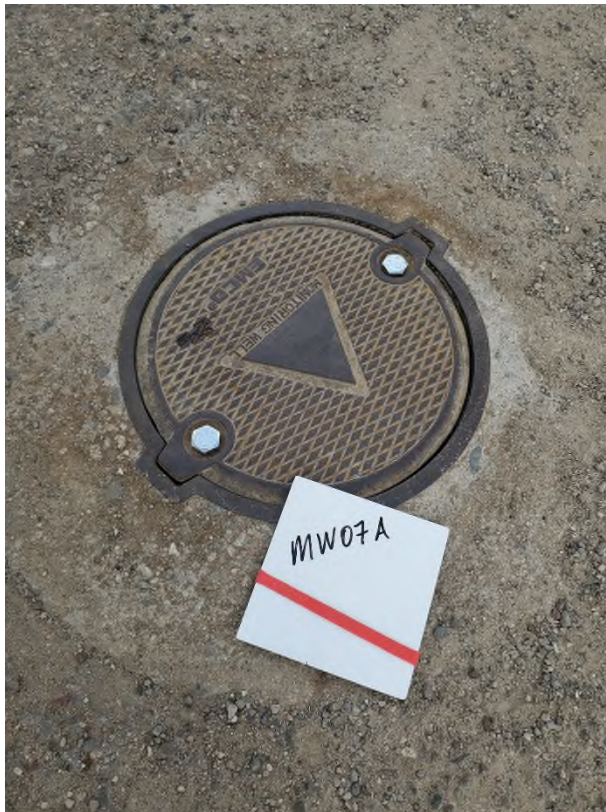
Photo #10: Condition of WR-MW-07A after well maintenance. Bolts were replaced.
