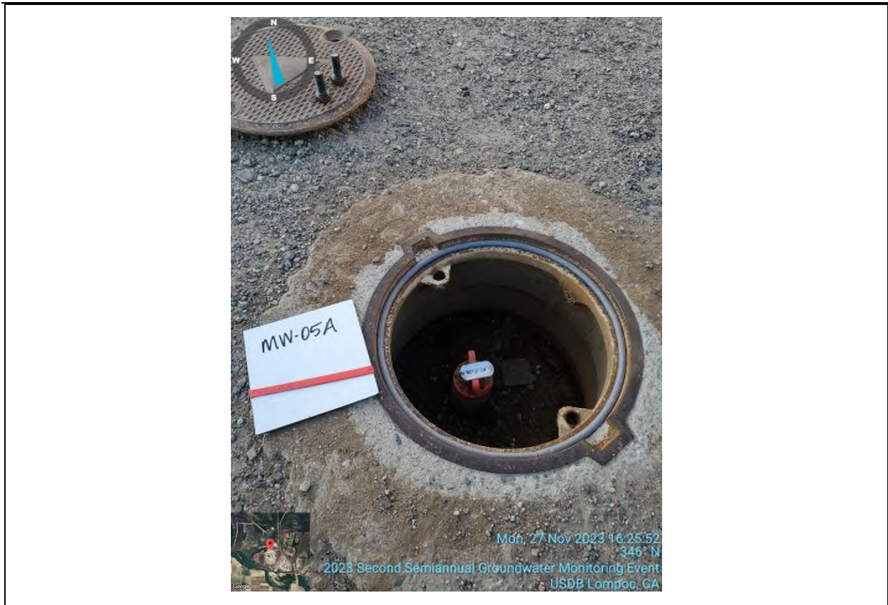
Photo #7: Condition of WR-MW-05A after well maintenance.
