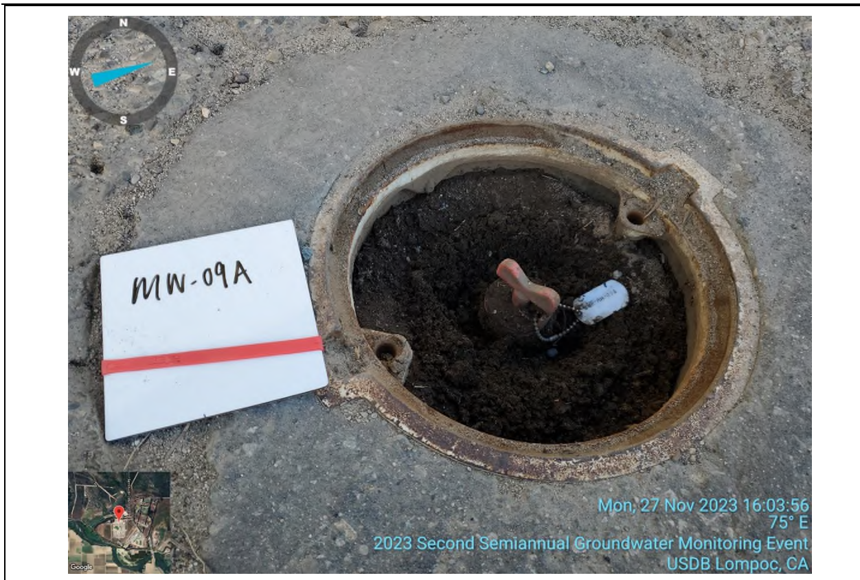
Photo #5: WR-MW-09A prior to well maintenance.
