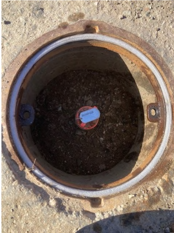
Photo #9: Condition of WR-MW-02 after well maintenance. Repairs were attempted on the well lid tabs but unable to re-thread sufficiently.
