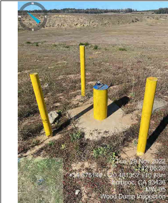
Photo 7: WD-MW-05 in good condition (facing northwest)
