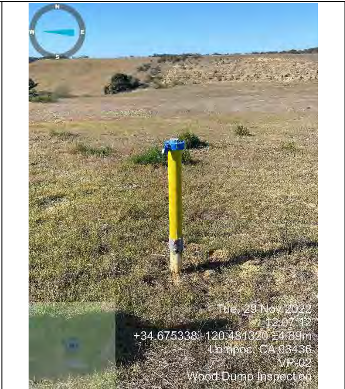
Photo 8: WD-VP-02 in good condition (facing west)
