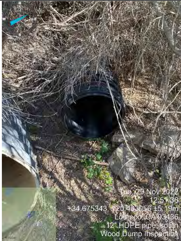
Photo 23: Southwestern Overside Drain Outlet – pipe is in good condition, but the opening is obstructed by vegetation and soil buildup (facing north)
