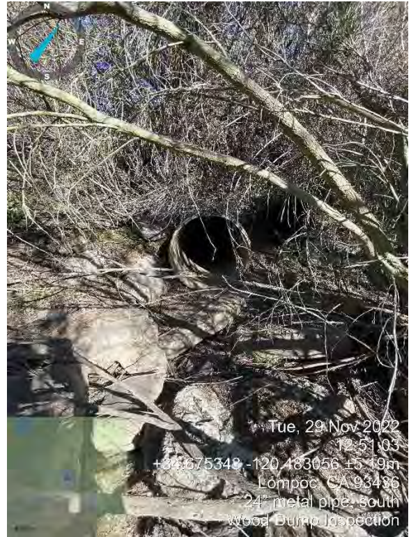
Photo 24: Southern Outlet of 24" Corrugated Metal Pipe – an area near the outlet is overgrown with woody vegetation, but the pipe is in good condition and unobstructed (facing northeast)
