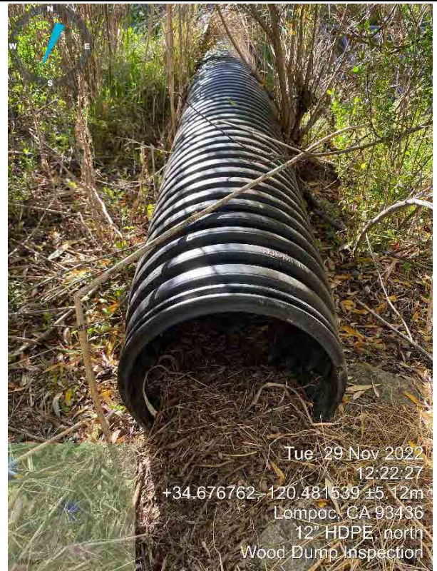
Photo 12: Northern 12" HDPE Drainpipe Outlet – pipe in good condition with minimal debris buildup at outlet (facing southwest)
