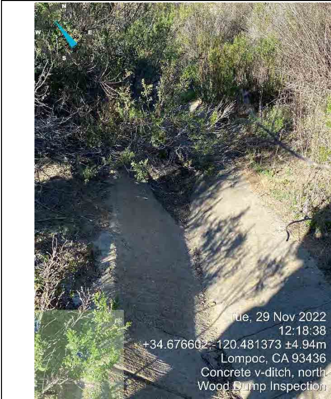
Photo 11: Northeastern Concrete V-Ditch – concrete in good condition, partially obstructed by soil and vegetation (facing northwest)
