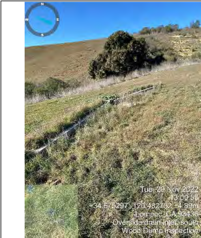
Photo 31: Southern Oversight Drain Inlet and Wingwall unobstructed and undamaged (facing northwest)
