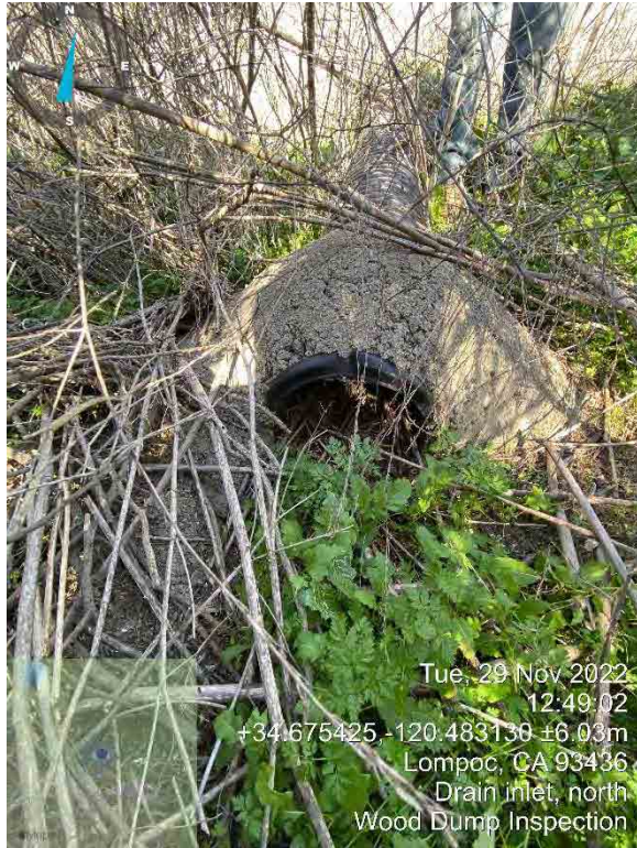
Photo 23: Southwestern Overside Drain Outlet – pipe is in good condition, but the opening is obstructed by vegetation and soil buildup (facing north)
