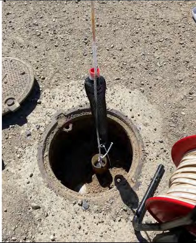
Description: Installing PDB at WR-MW-08A.
