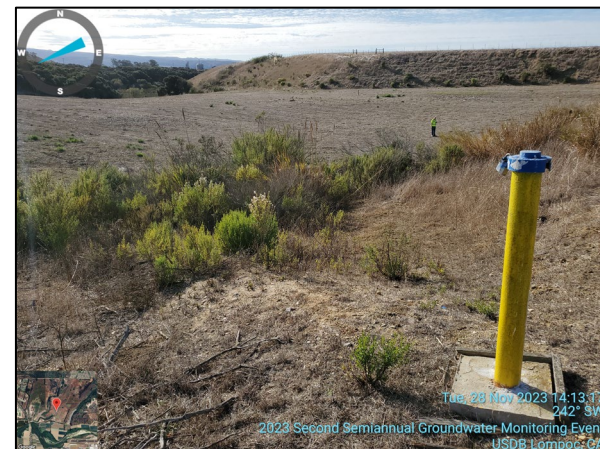
Vapor Probe (WD-VP-01) in foreground, Wood Dump cover in background
