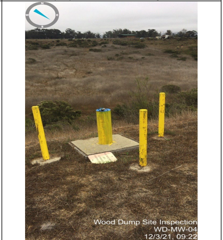
Photo 20: Groundwater monitoring well, WD-MW-04, facing southeast.
