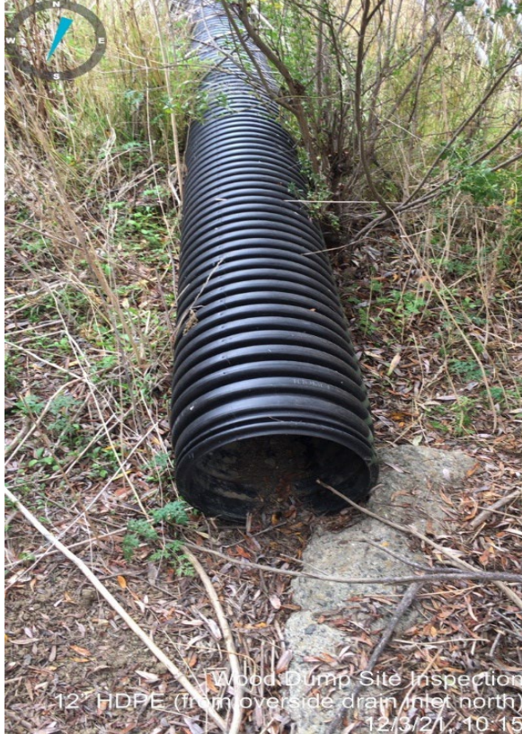
Photo 5: 12-inch HDPE drainpipe (north side of Site), facing southwest.
