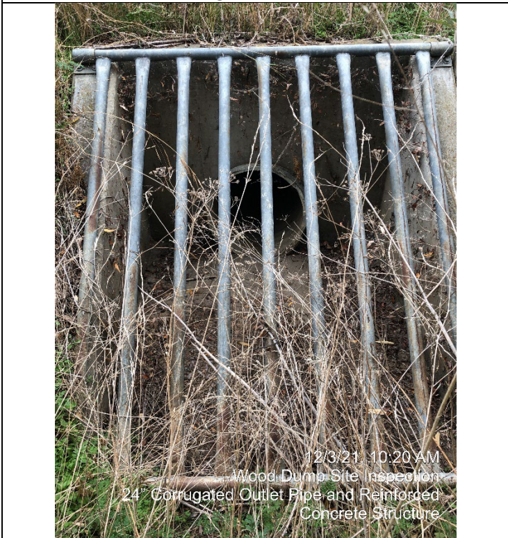
Photo 3: 24-inch corrugated outlet pipe and reinforced concrete structure (north side of Site), facing south.
