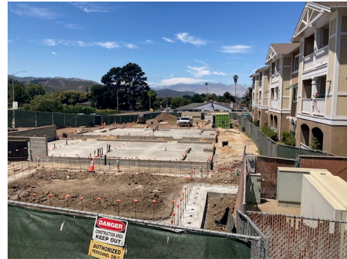
Site During Construction
