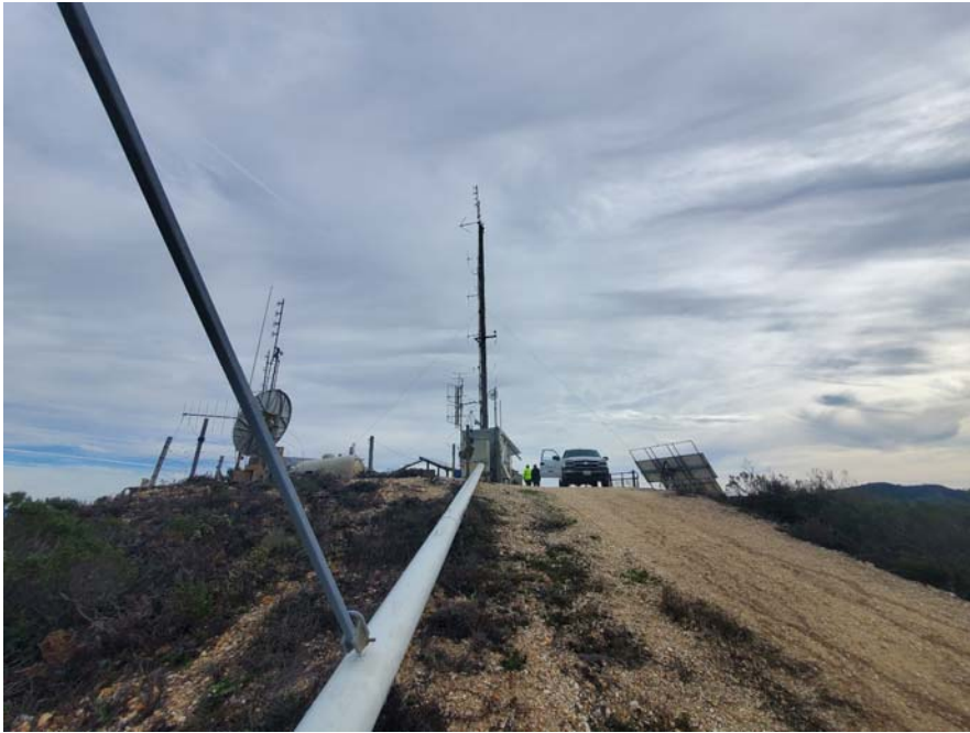
Notes: North to south view of site.
