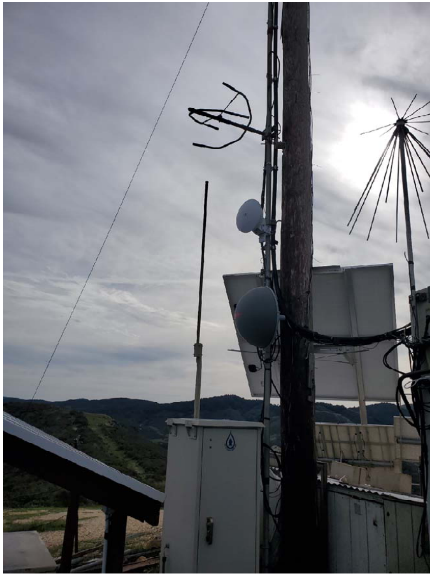
Notes: Ubiquiti second antenna from the top Scada/ LMR on the link.
