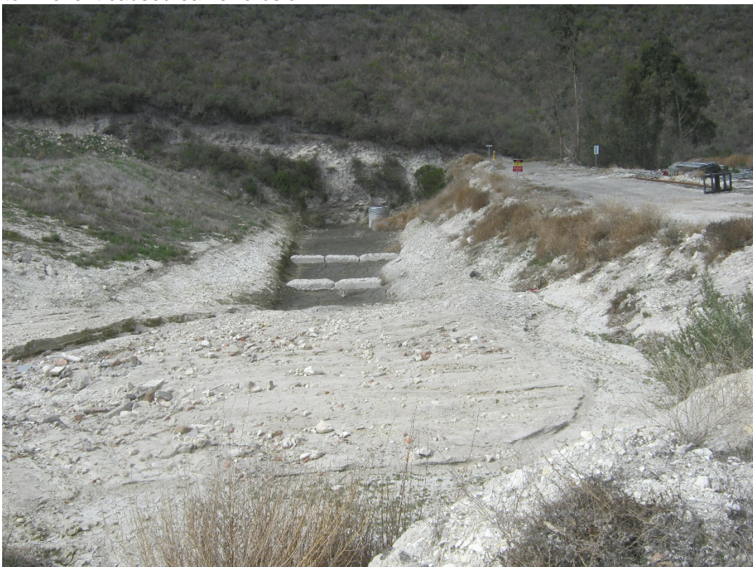
Photo 4 – Sedimentation basin shown in Photo 3 taken on February 22, 2018 after January 9, 2018 storm event caused earlier erosion.
