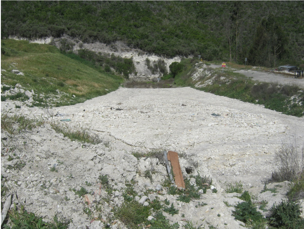
Photo 4 – Sedimentation basin shown in Photo 3 taken on February 22, 2018 after January 9, 2018 storm event caused earlier erosion.
