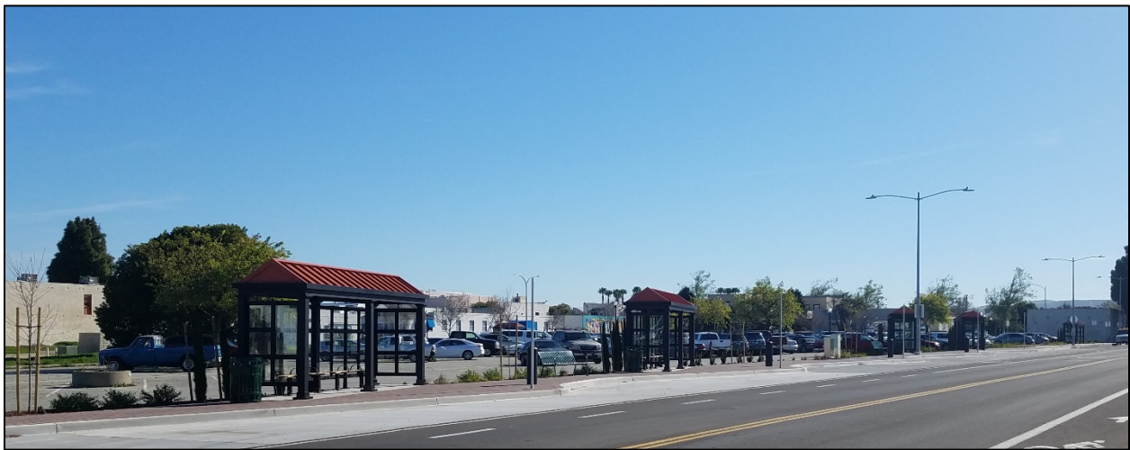
Figure 4 - Transit Transfer Center, City of Lompoc
