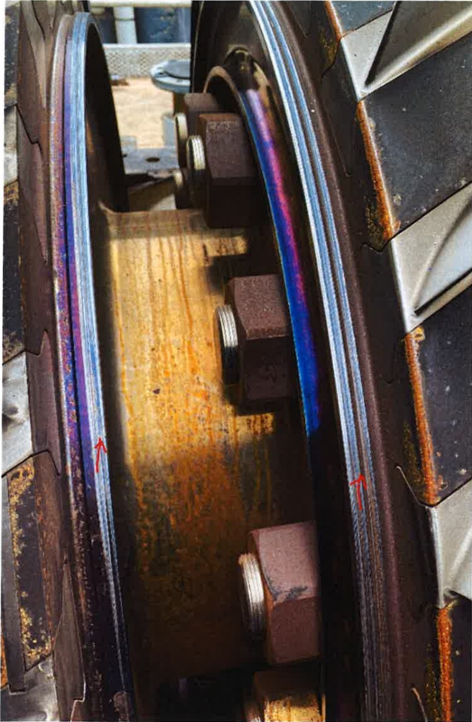
Seals have been bent over and smashed.
