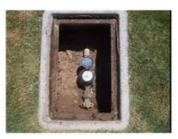
The meter is usually in a plastic or cement rectangular box flush to the ground with a small hole in the top of the box, normally located close to the street and/ or sidewalk or alley close to your property line. The number of the meter should match the meter number on your water bill.
