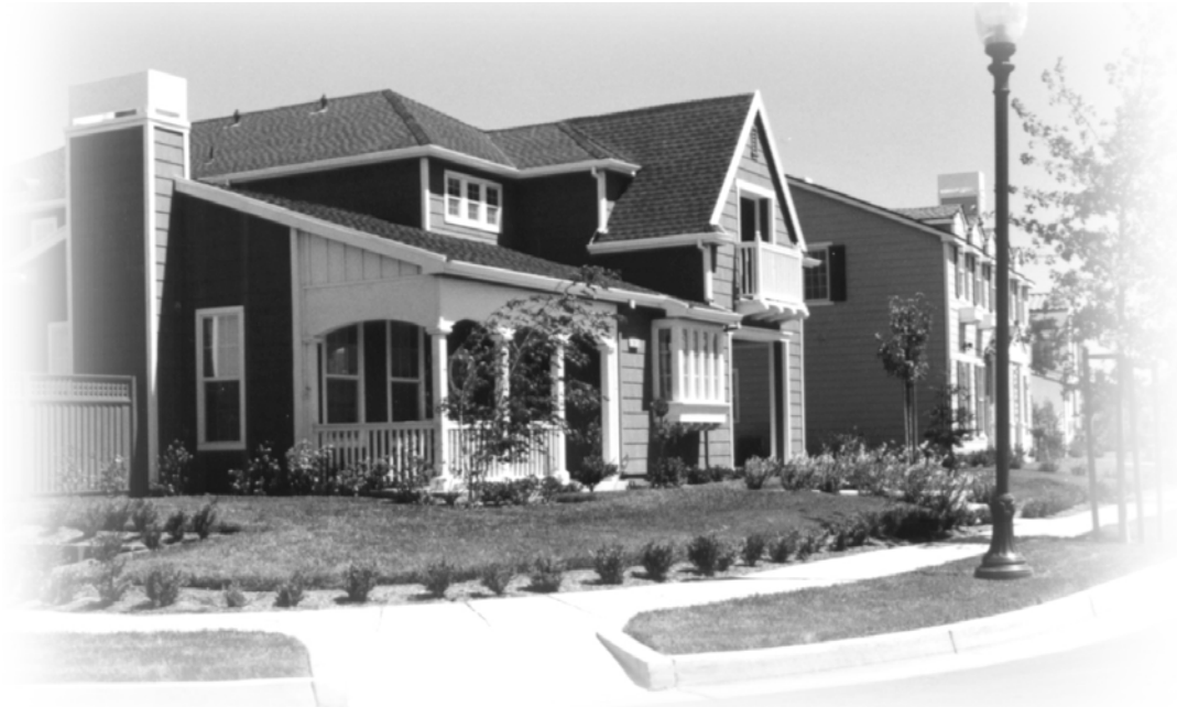
Figure 34 – Example of Well-Executed Massing
