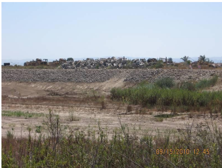
Photo 6 - Rock Rip-Rap Bank Protection – Santa Maria River near Suey Crossing
