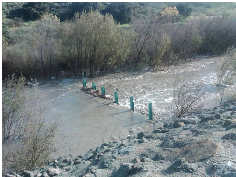
Photo 2 - Arroyo Simi, January 2010 just after construction
