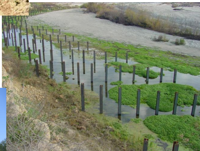
Photo 9 - Same location immediately after pile installation (2002)
