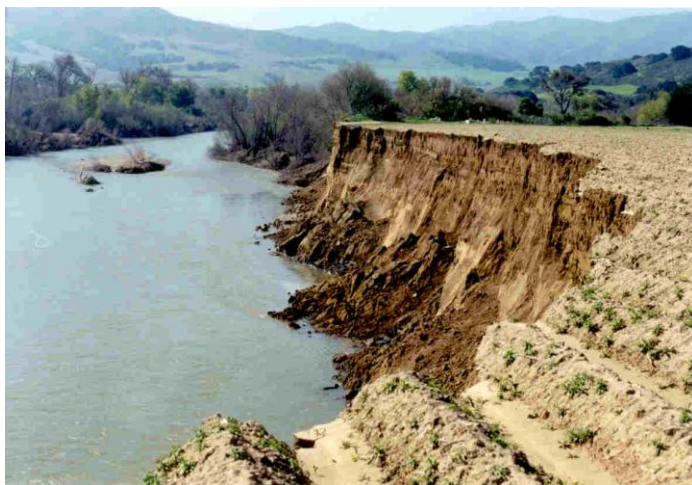
Photo 7 - Storm damage on Santa Ynez River 2001
