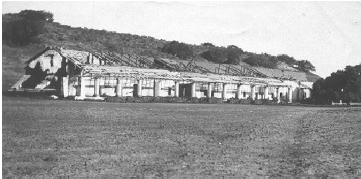
Early 1900's, post fire and pre-ruin state of the residence building.
