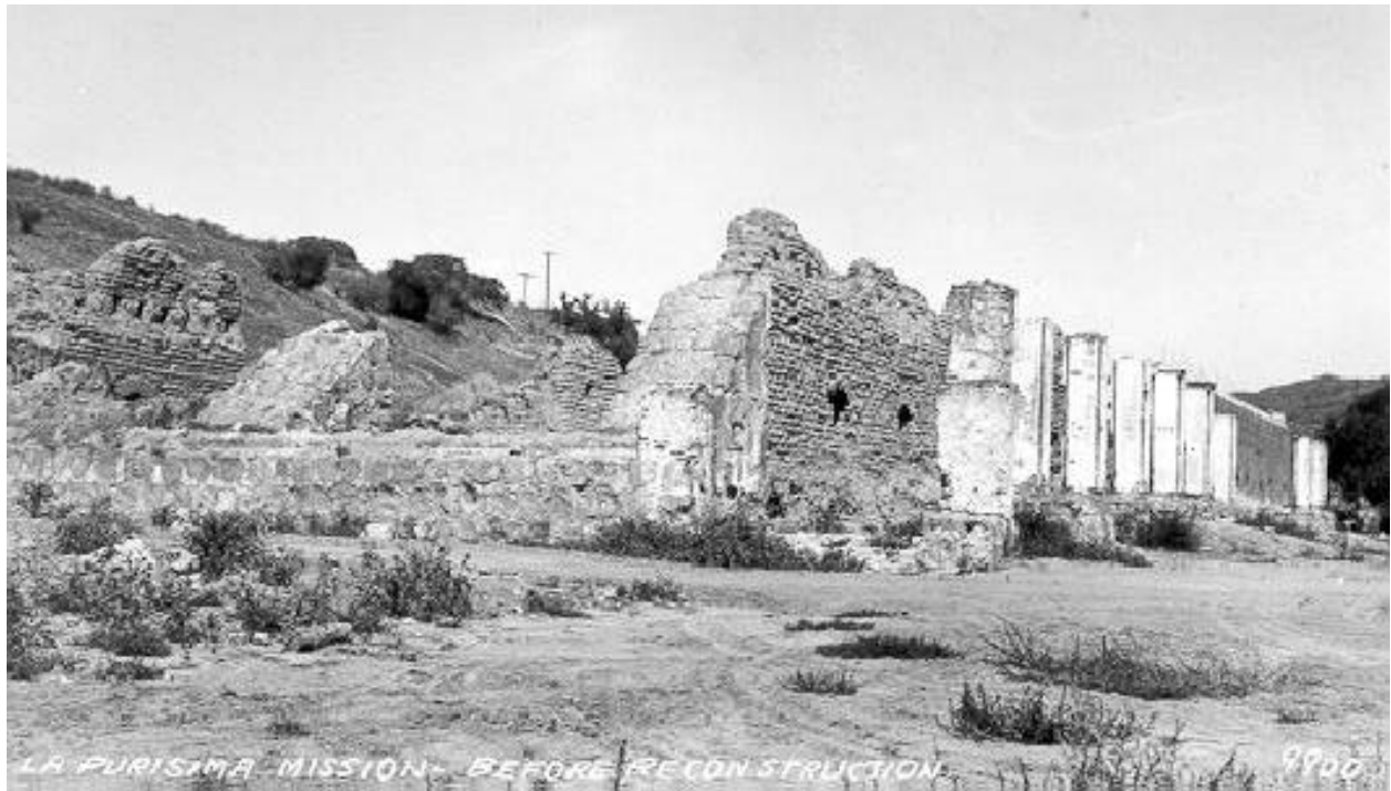
Early 1930's, final stage of dilapidation prior to restoration.
