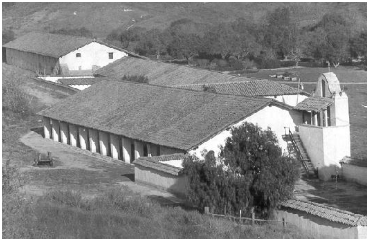
The backside of the Mission, looking down from the hillside.
