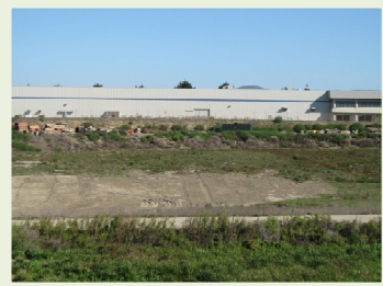
S4 - Drying bed: aged sludge is pumped from the lagoons to the drying bed where sludge dries.
