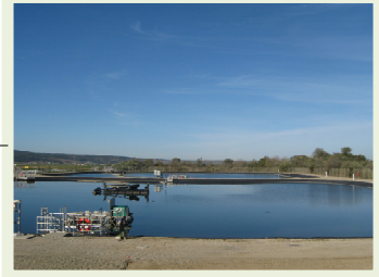
S3 - Lagoons: location where digester sludge is pumped to age for one year.
