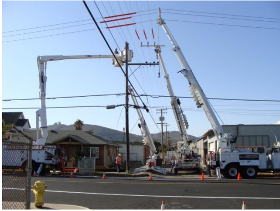
4-kV to 12-kV Line Conversion
