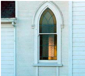
Constructed in 1888, the First Baptist Church on West Cypress Avenue is one of Lompoc's earliest churches.
